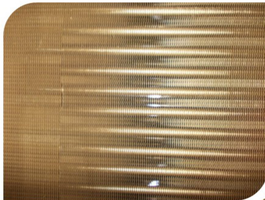
GAS COOLER AFTER COATING
