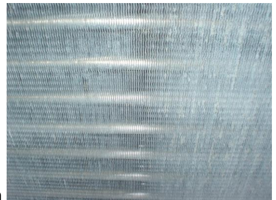
After Deep Clean
