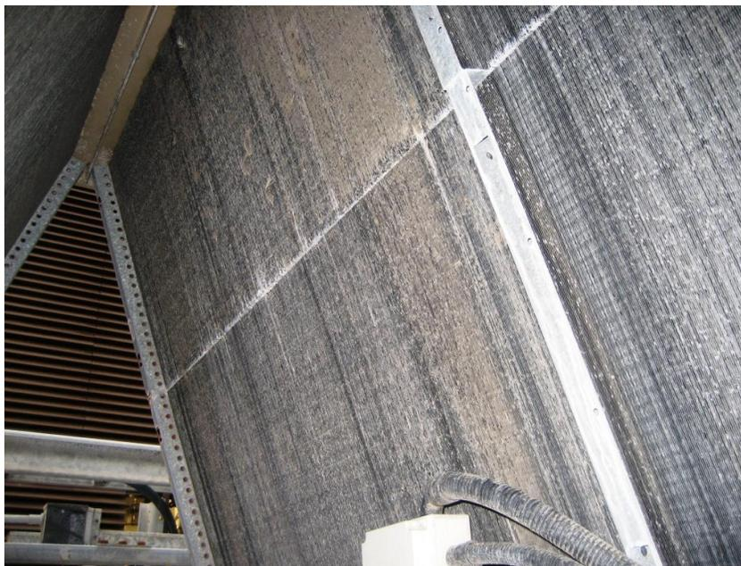
The coating was applied on site, situated on the roof. The fan covers were removed during cleaning and the blades were dismantled during coating to allow access from the top to the inside surfaces of the coil.
